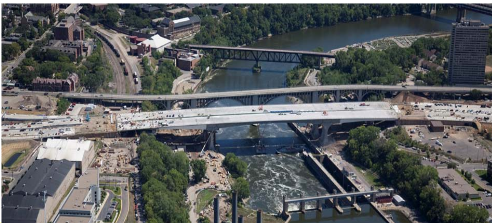
Bridge complete in 339 days, 3 months ahead of schedule.
