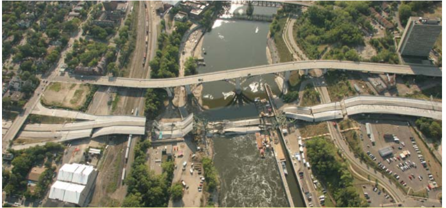
The St. Anthony Falls Bridge Collapsed on August 1st, 2007
